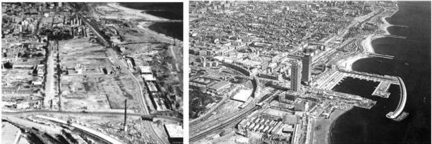
Fig 3 | Illustrates the dramatic transformation of Barcelona's coastal front. The left panel depicts the area under construction in 1990, with vast brownfield sites being prepared for development. The right panel, taken in late 1991, shows the nearly completed Olympic Village, which not only provided facilities for the Olympics but also permanent housing and recreational spaces for residents, catalyzing a significant boost in local tourism and enhancing the city's global image
